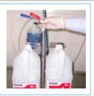
Undo cap on new bottle and carefully place in feed pipe
