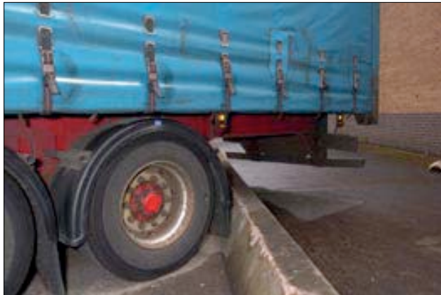
Figure 7 Concrete wheel stop
